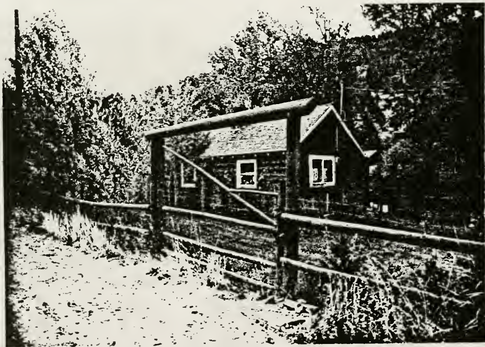
Figure 57. Structure complex #12, log house, south end.
